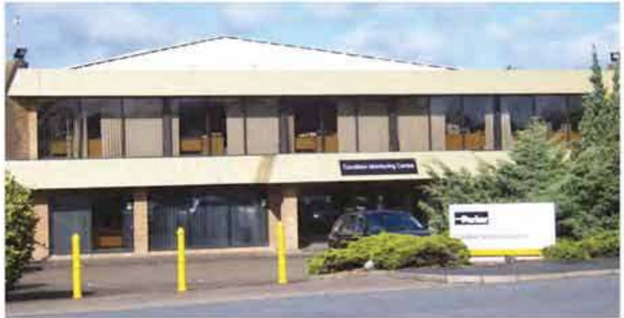
Condition Monitoring Business Unit, Thetford, UK
