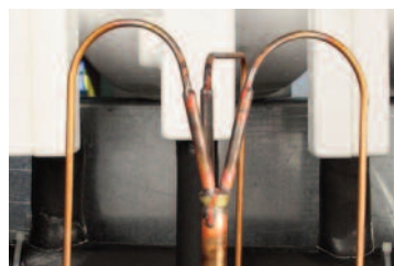
Expansion Device-Capillary
